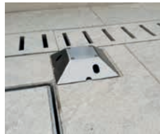
Vehicle-resilient photocells
